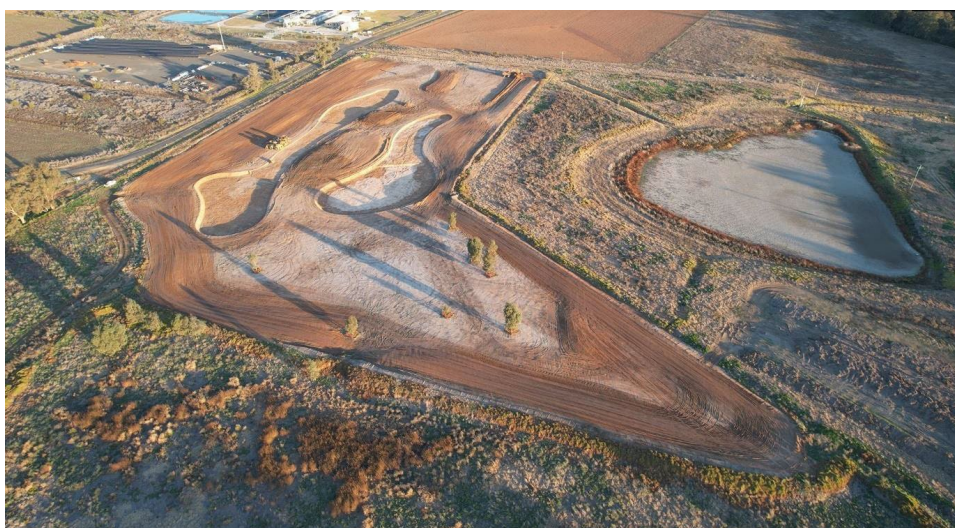
May 2023 - Major earthworks complete.
